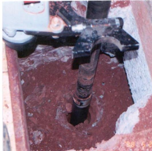
Rock drilling operation adjacent to the structural wall. Notice that the footing is notched to allow the pier to be installed as close as possible to the wall load. The entire installation takes place in an excavation not larger than 3 feet square.
