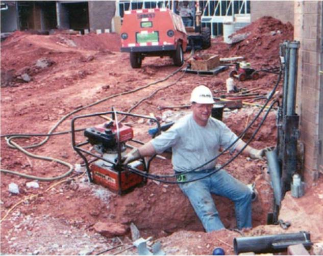
Here, a technician uses quiet, vibration-free hydraulic equipment to install an Atlas Resistance® Pier.
