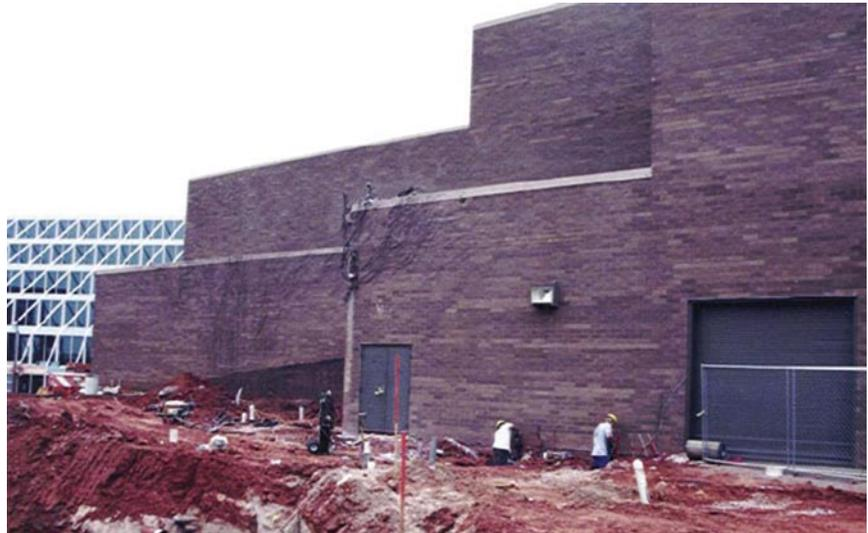
Above is a view of the job site where workers are installing supplemental support. Atlas Resistance® Pre-Drilled Piers provided support to the existing structure during excavation.
