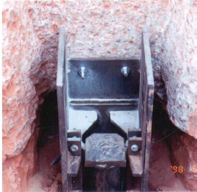
Close-up view of the installed pier. The Atlas Resistance® Pre-Drilled Pier System is constructed of 1/2" and 3/4" steel for heavy-duty applications. The assembly weighs nearly 300 pounds and has an ultimate capacity of 76,000 pounds!
